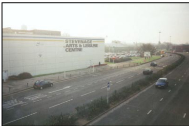
Six lanes of traffic along Lytton Way.
