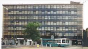
Existing view of Council Building
