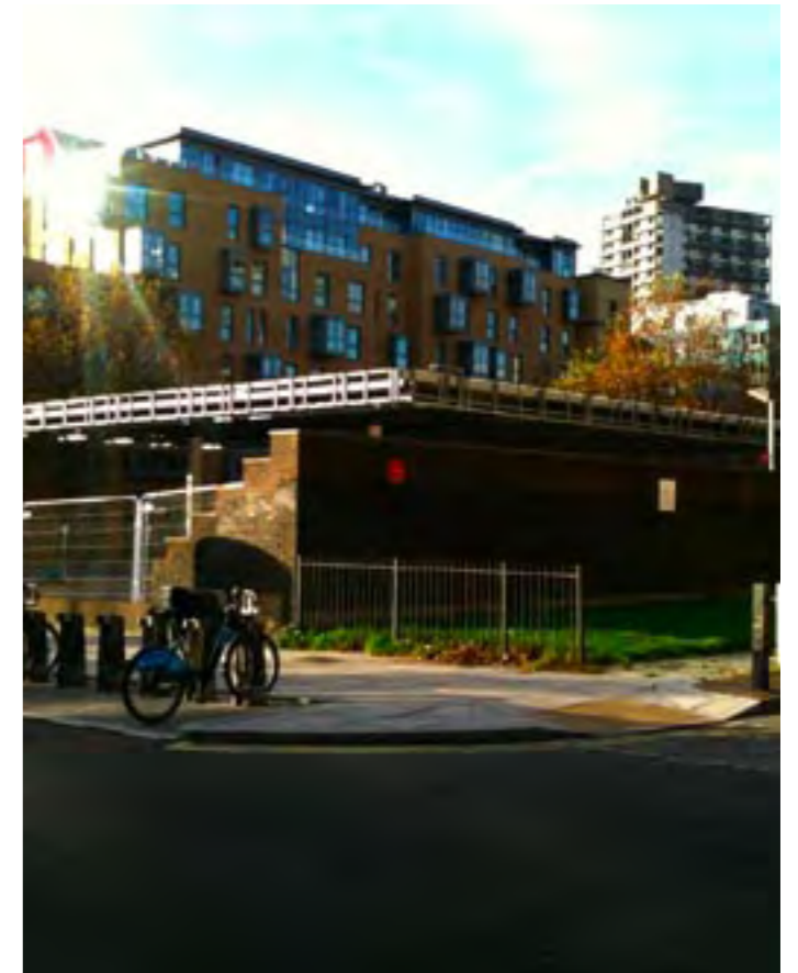
Garage Site, Walworth Road
