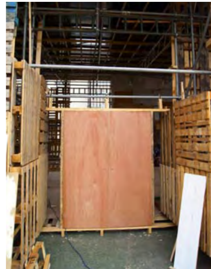
The Oikos Project under construction www.oikosproject.com/ Image: Ed Fyfe
