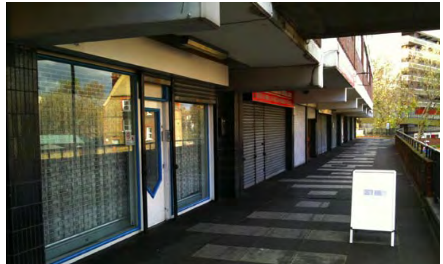
The Parade of Units, The Club Building on Rodney Place
